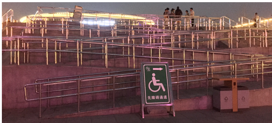
Figure 5 – User-unfriendly design of barrier-free access facilities
